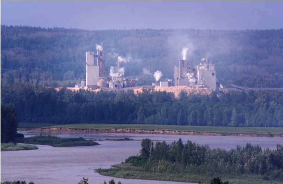
Pulp mill along the Fraser River at Prince George.
